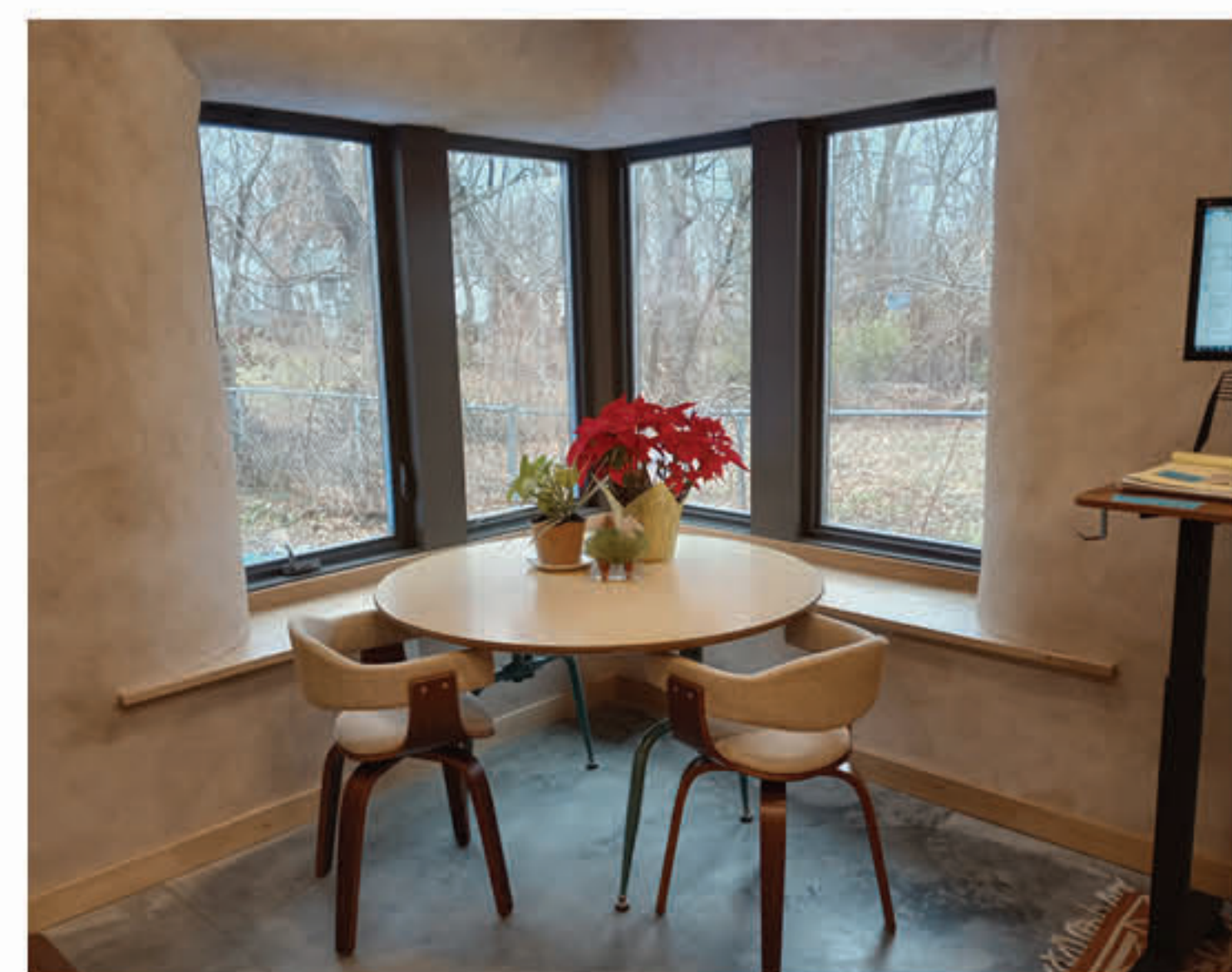
A CLOSE-UP OF THE DINING AREA. NOTE THE INSULATIVE, THERMALLY MASSIVE STRAW BALE WALLS, MOST APPARENT IN THE WINDOW WELL. PHOTO COURTESY OF ADRIENNE STOLWYK.
