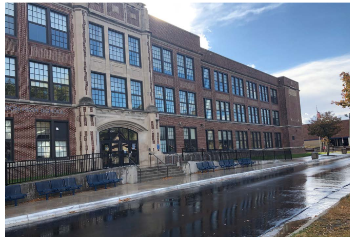
EDISON HIGH SCHOOL IN MINNEAPOLIS. PHOTO BY CONNOR ARNESON
