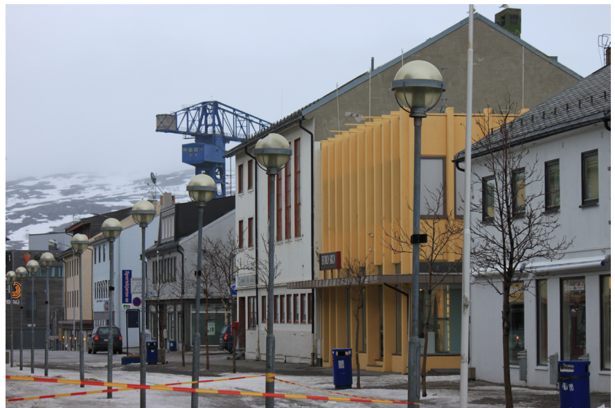
"AFTER TARGET PRACTICE." KIRKENES, NORWAY. DESTROYED BY RUSSIAN BOMBS DURING WWII, IT'S A PRAGMATIC POST-WAR REBUILD.
