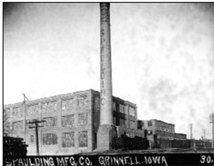
Figure 6: Spaulding Factory Building #5 from SW (Courtesy Drake Community Library)
